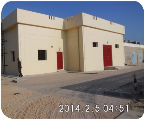
SWITCH GEAR ROOM – CENTRAL SALALAH
