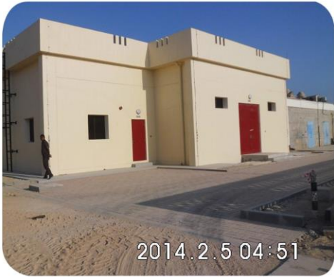
SWITCH GEAR ROOM – CENTRAL SALALAH
